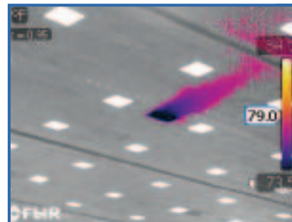
Facility AC vent cycling air in the incorrect direction.
