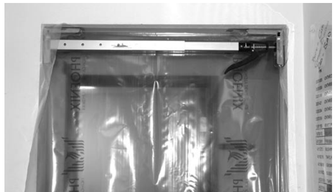
Figure 3: Properly installed Phoenix Quick chamber
